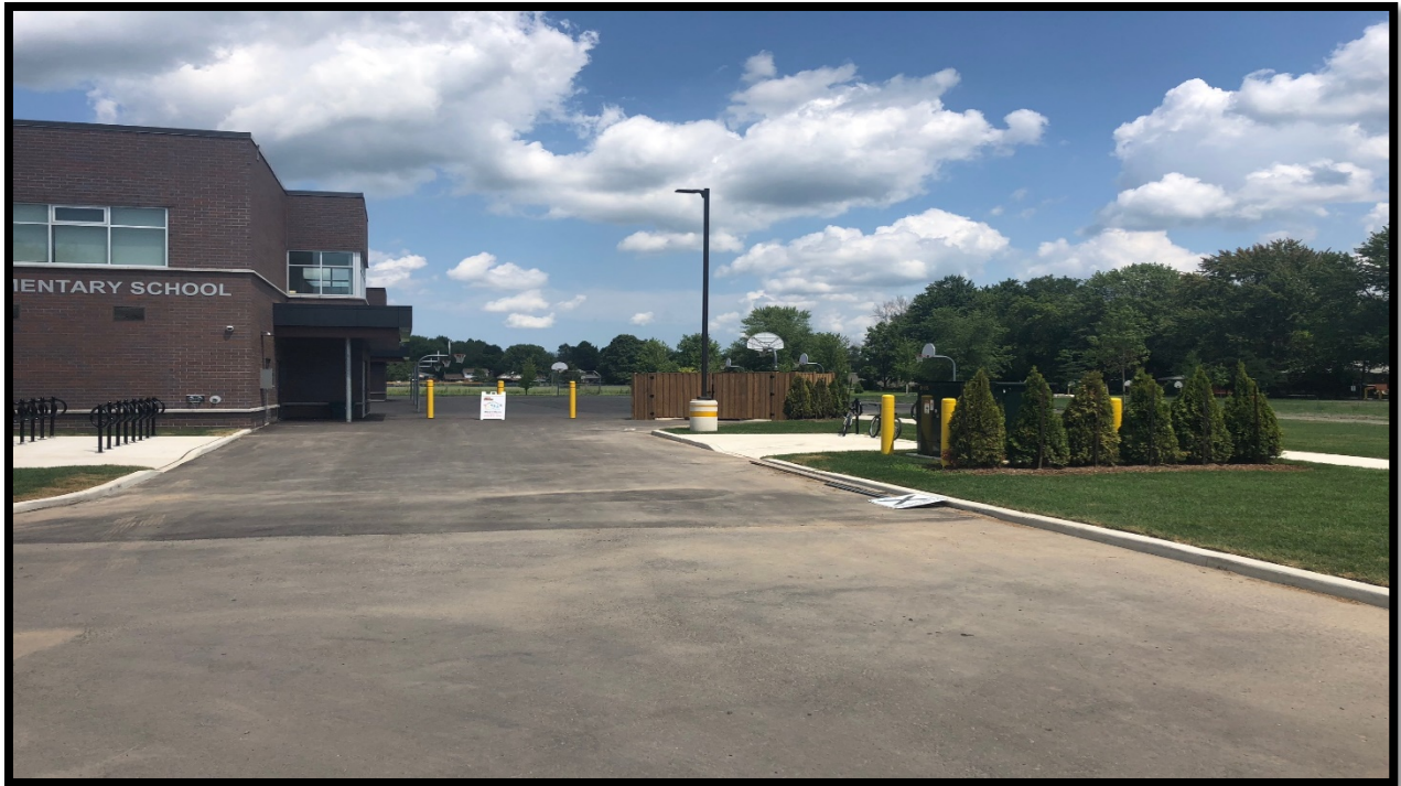
Site Work - Completed
