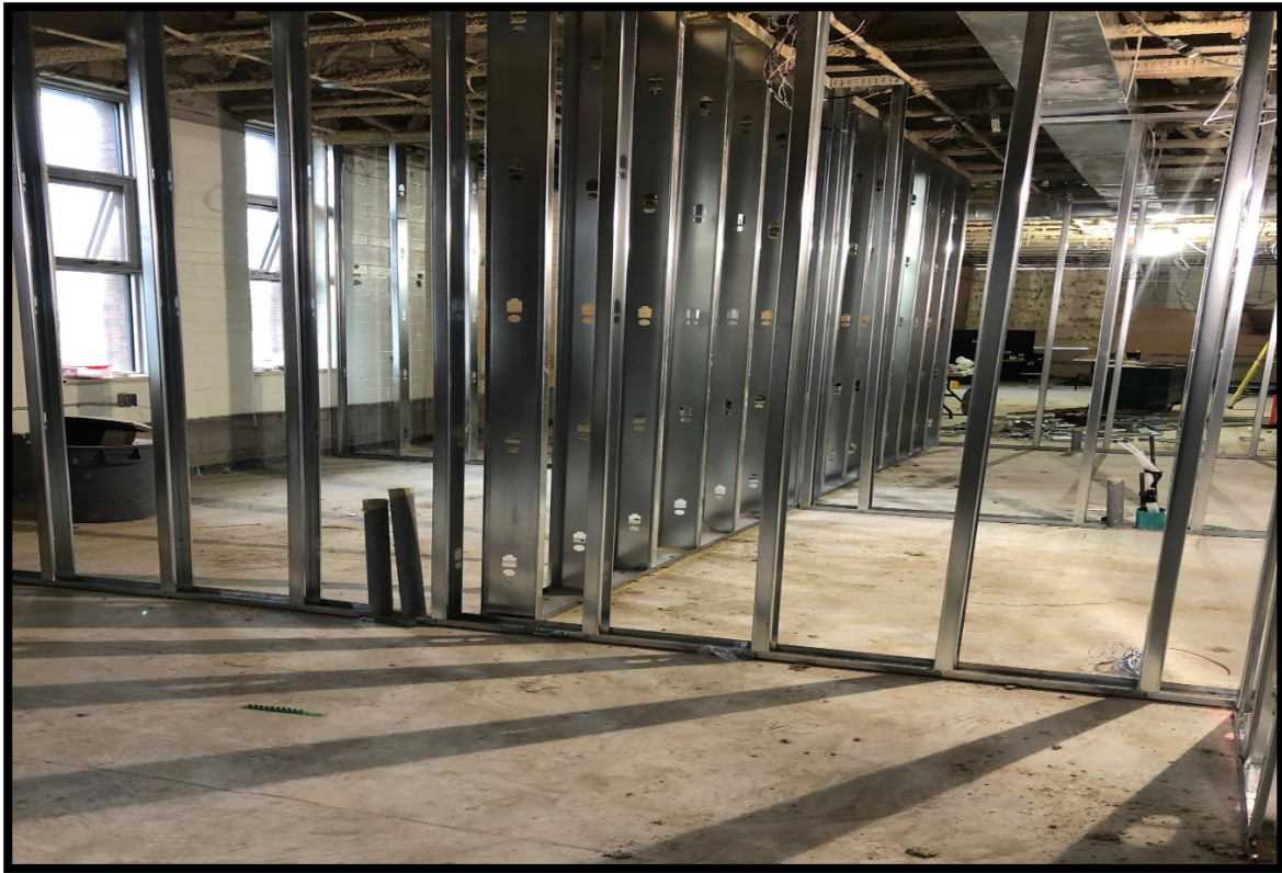
Figure 1: Internal Wall Construction at Hagersville SS
